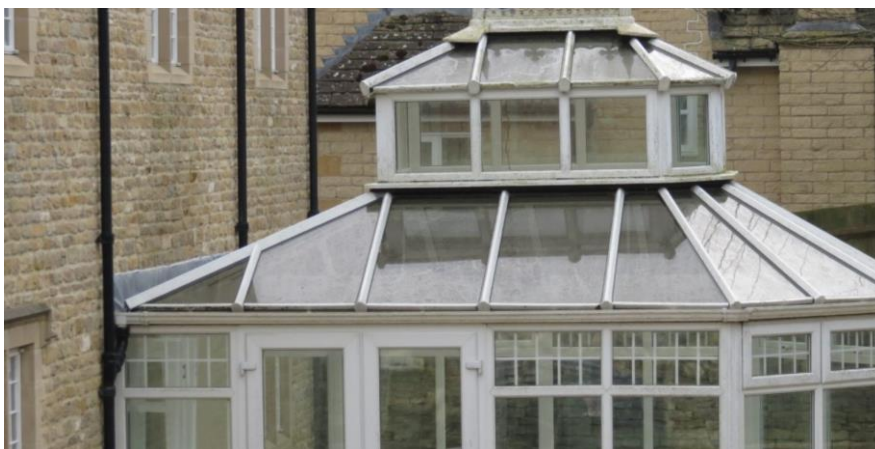
Figure 4 – uPVC rear conservatory at 19 Old North Road
